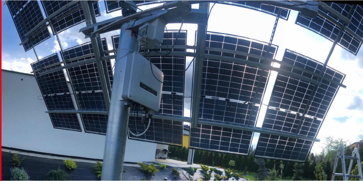
Residential PV Project in Poland
