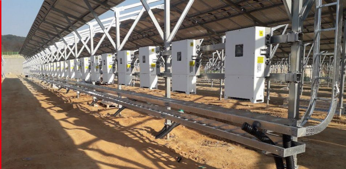
PV Power Plant in Korea
