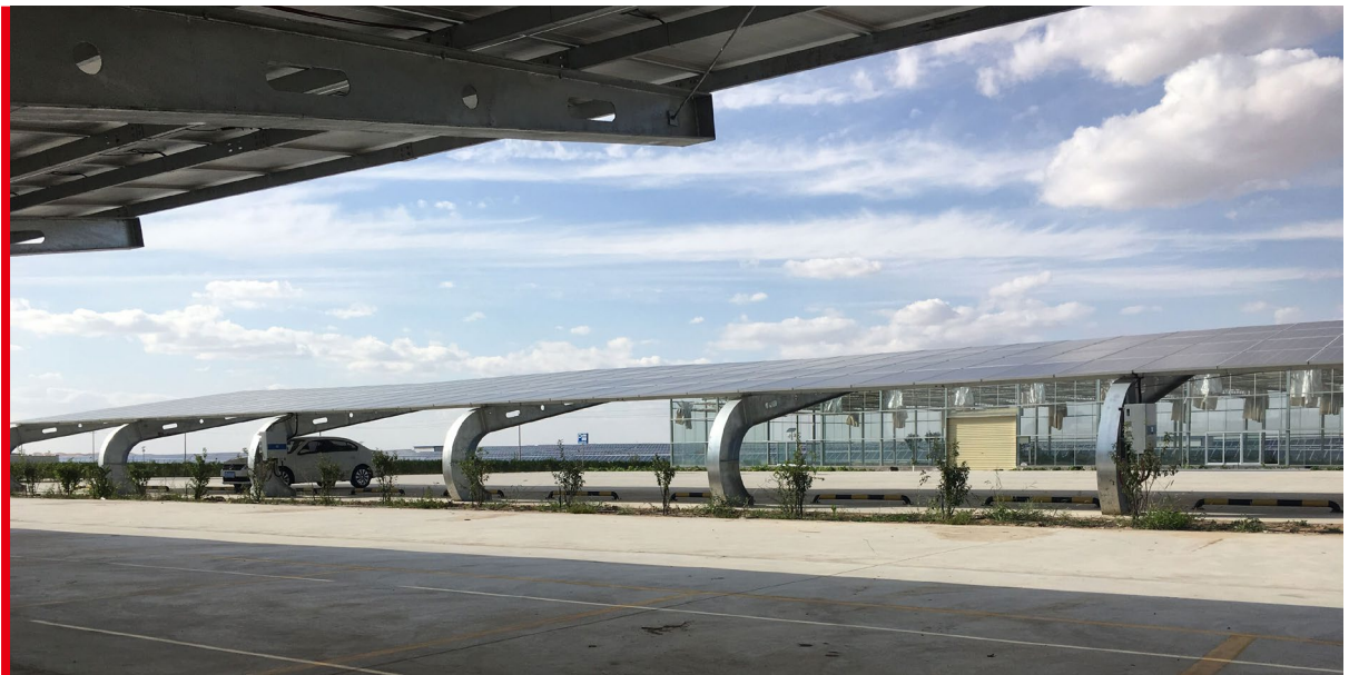
Distributed PV Power Station for the Parking in Ningxia, China
