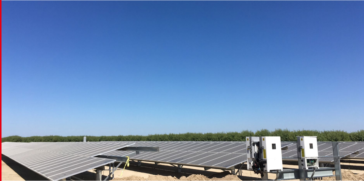
Distributed PV Power System for the Farm in Madera, USA
