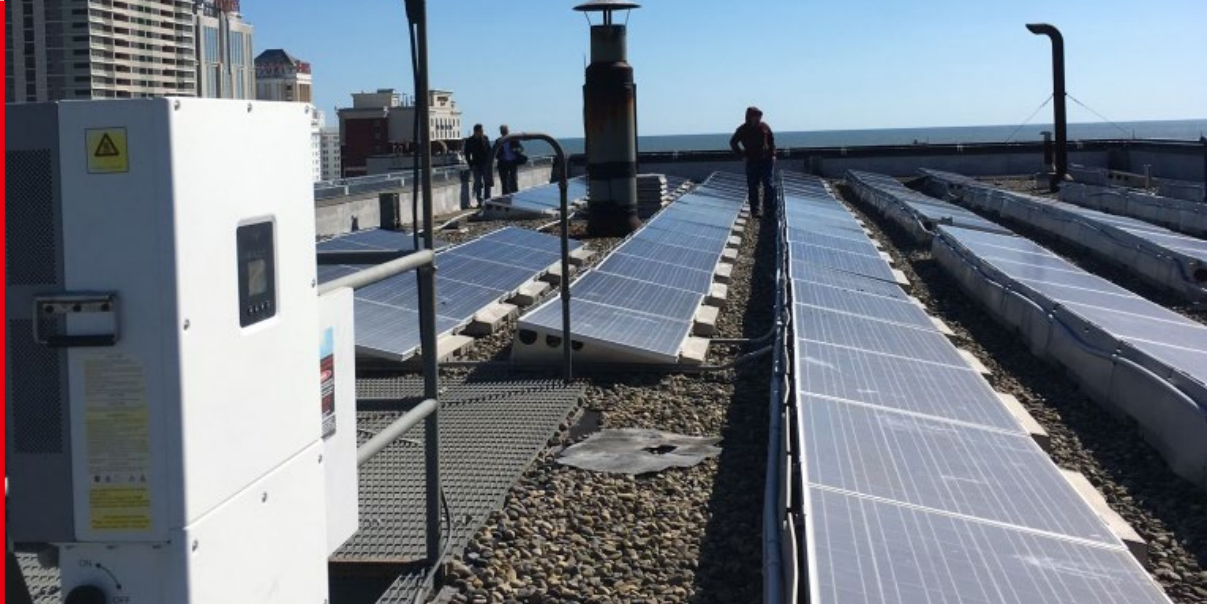
Atlantic County Government Office Rooftop System in New Jersey, USA
