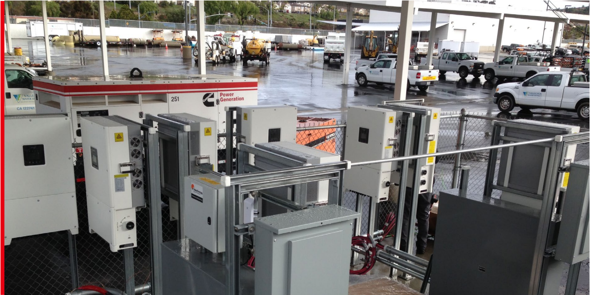
Distributed PV Power Station for the Parking in San Marcos, USA
