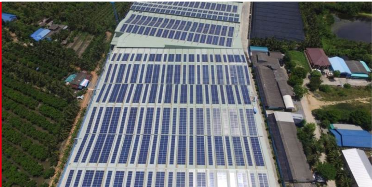
2MW Rooftop Distributed PV Power Plant of Factories in Bangkok, Thailand
