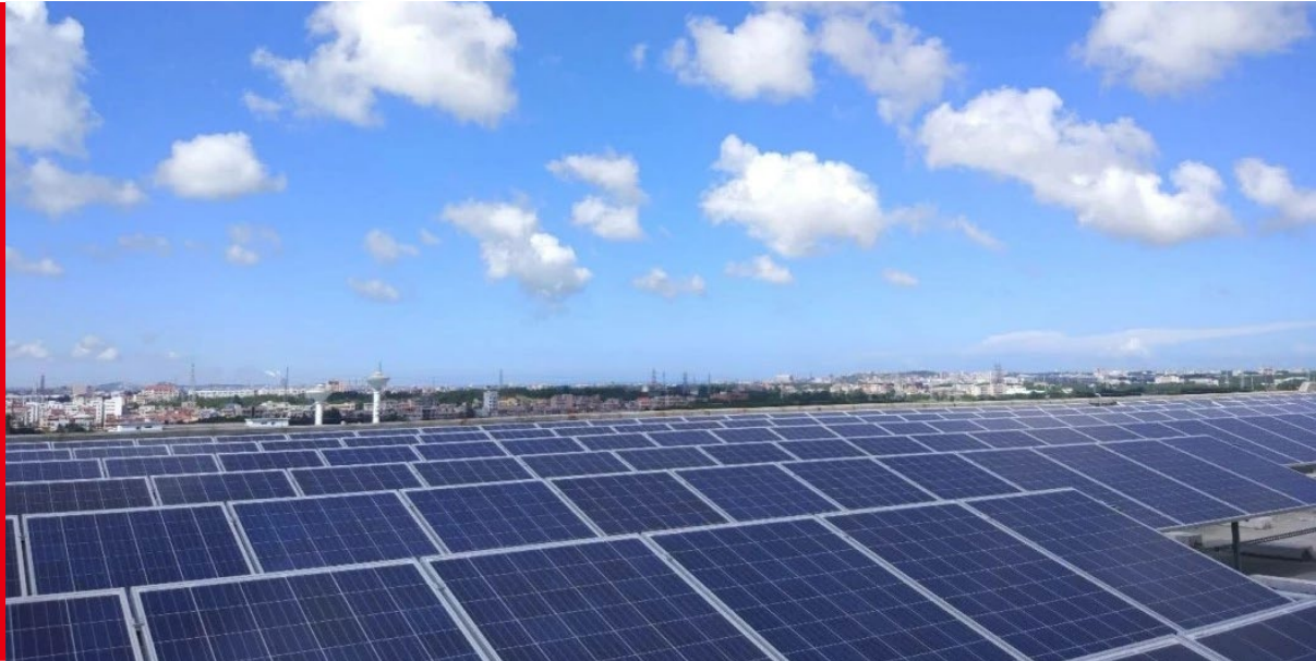
Jinjiang Jinjing Town Factory Roof Project, China
