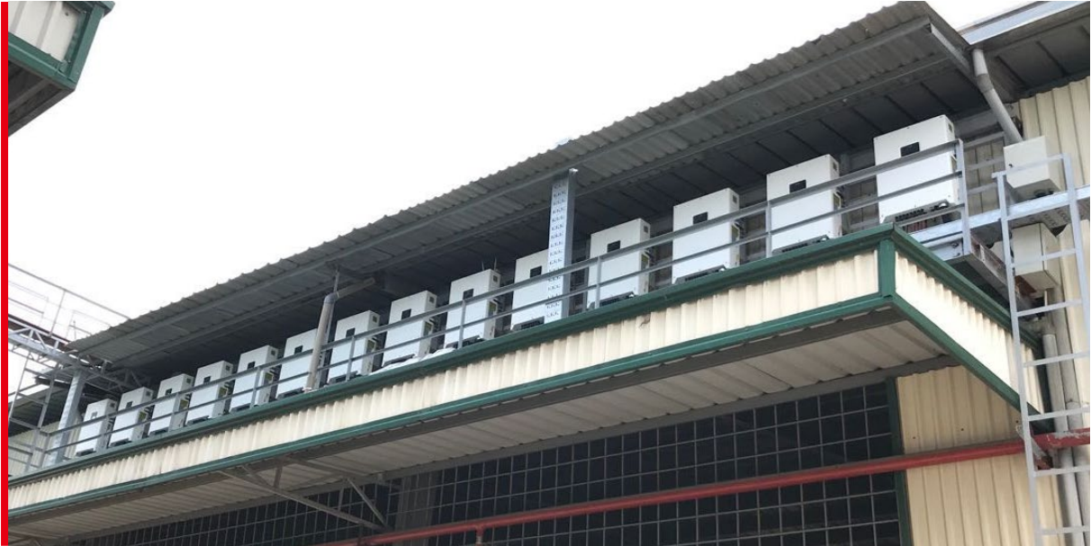
1MW Roof Distributed PV Power Station Project in Vietnam
