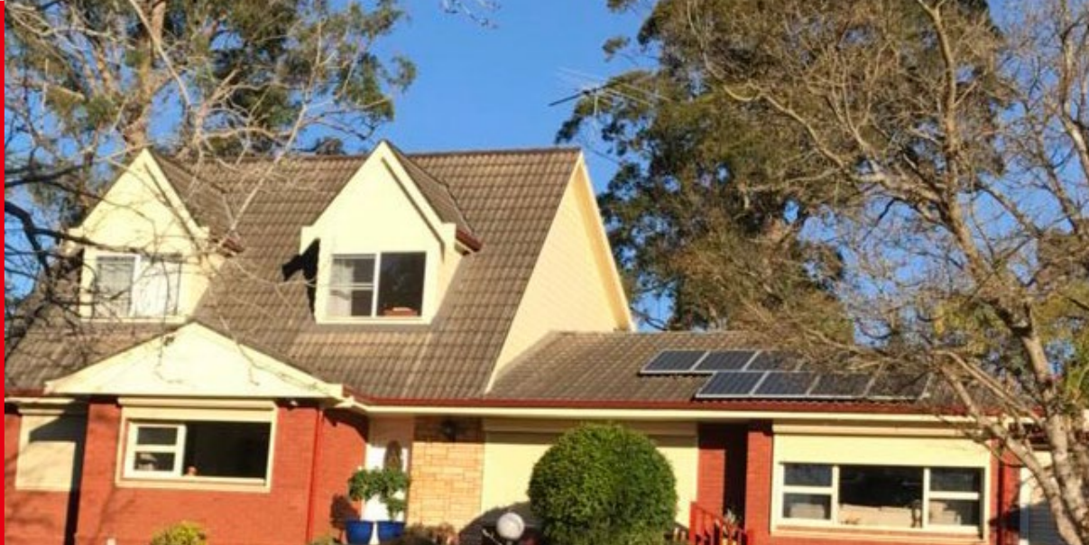
Residential Rooftop PV Project in Australia
