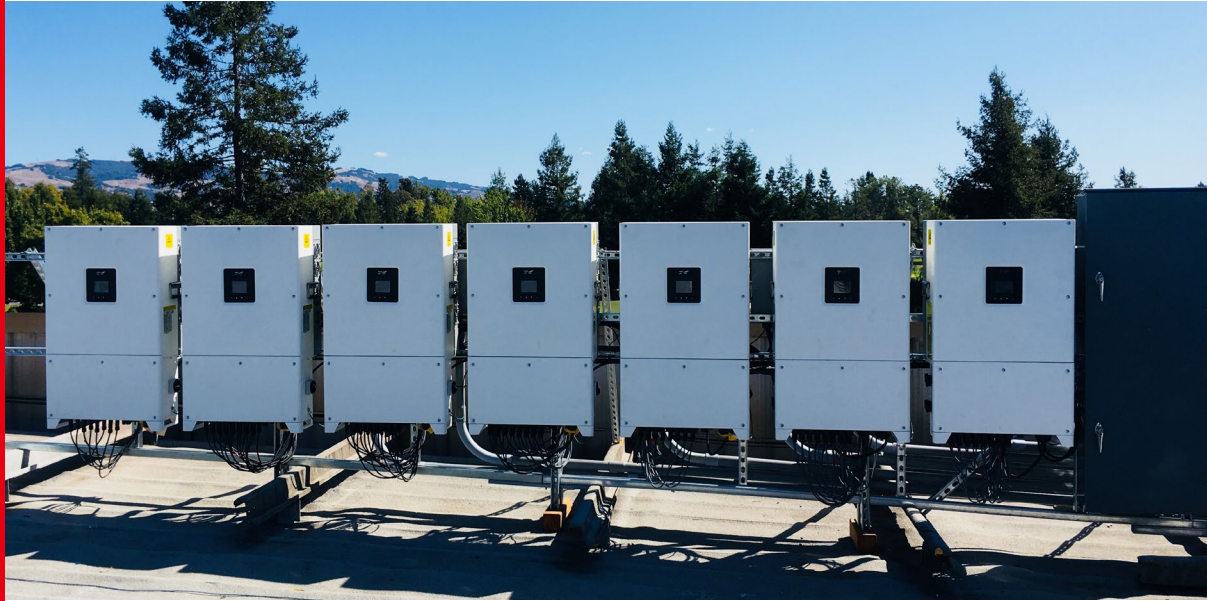
Double Decker Rooftop PV Project in San Francisco, USA
